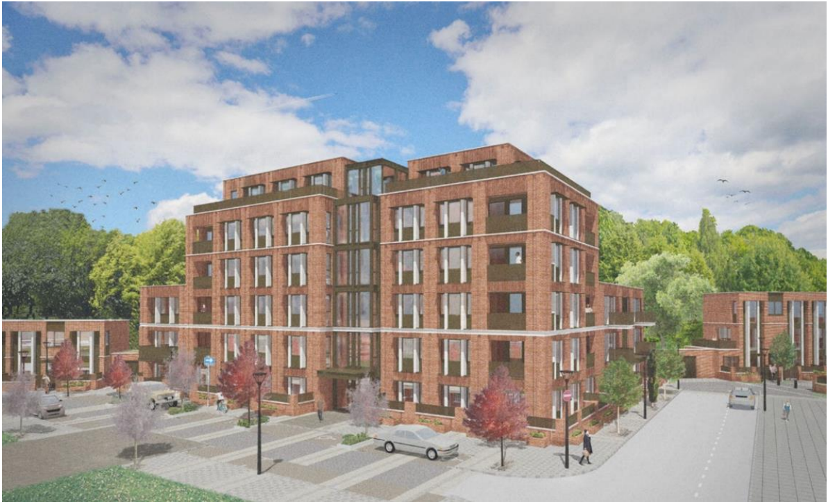
46 Council homes at Remington Road, Seven Sister starting on site March 2022 – fourteen with three-bedrooms and four with four-bedrooms, and five fully accessible for wheelchair-users
